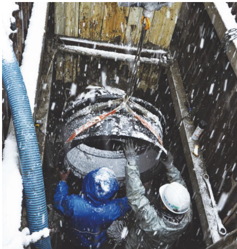
Photo 1: Repair of water distribution pipe with a diameter of 800mm [4]
