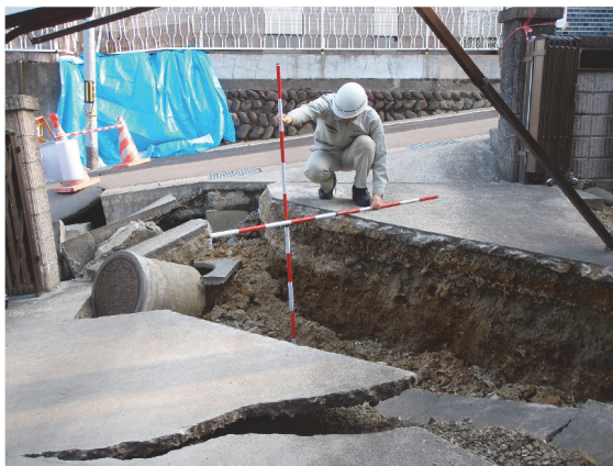
Photo 3 Large crack due to landslide in Midorigaoka (courtesy of Sendai City) Photo 4 Collapse of retaining wall in Asahigaoka
