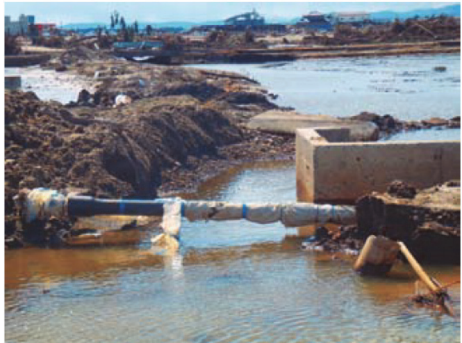
Photo 2: Earthquake-proofing water pipe with a diameter of 150 mm survived the tsunami [4]
