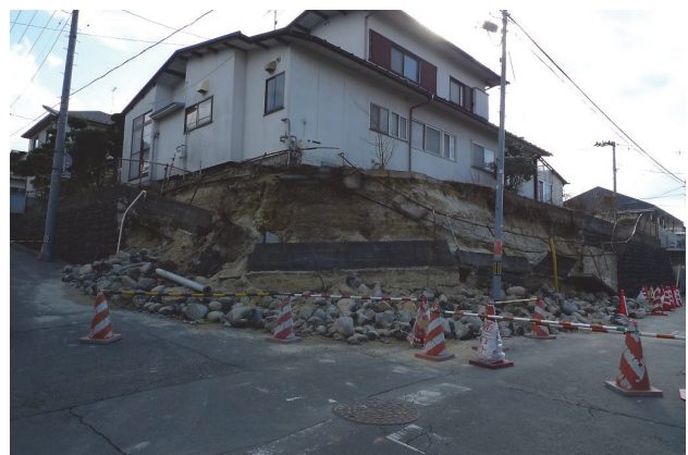
Photo 3 Large crack due to landslide in Midorigaoka (courtesy of Sendai City) Photo 4 Collapse of retaining wall in Asahigaoka
