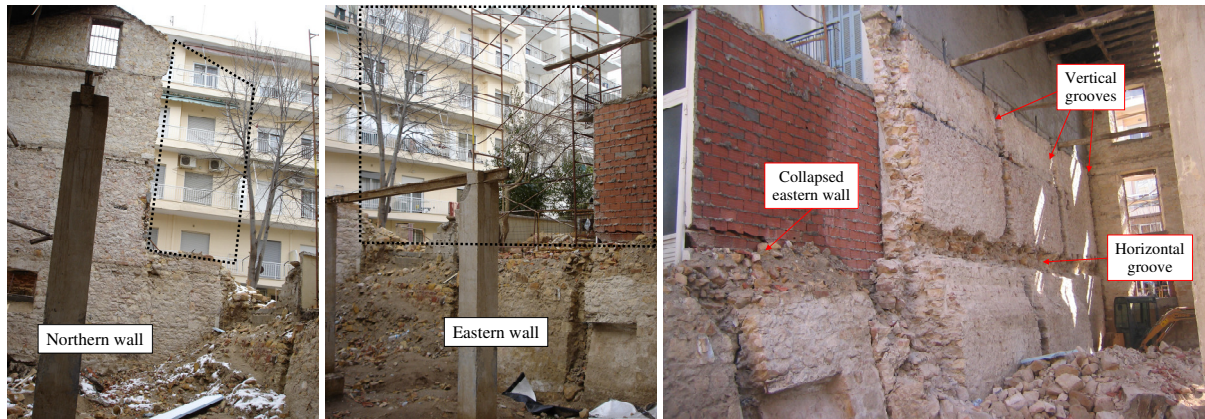
Figure 5: Inner views of the (a) northern and (b) eastern masonry walls of the building after the partial-collapse of 2005. (c) Eastern masonry has three vertical grooves and one horizontal groove on the internal part of the wall.
