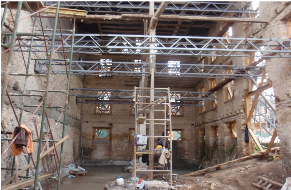
Figure 7: Inside view of the temporary supporting system of the substantially damaged eastern masonry wall.
