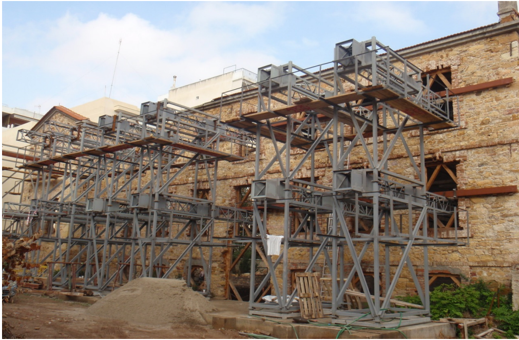
Figure 6: Outside view of the external non-permanent steel towers for the temporary support of the façades.
