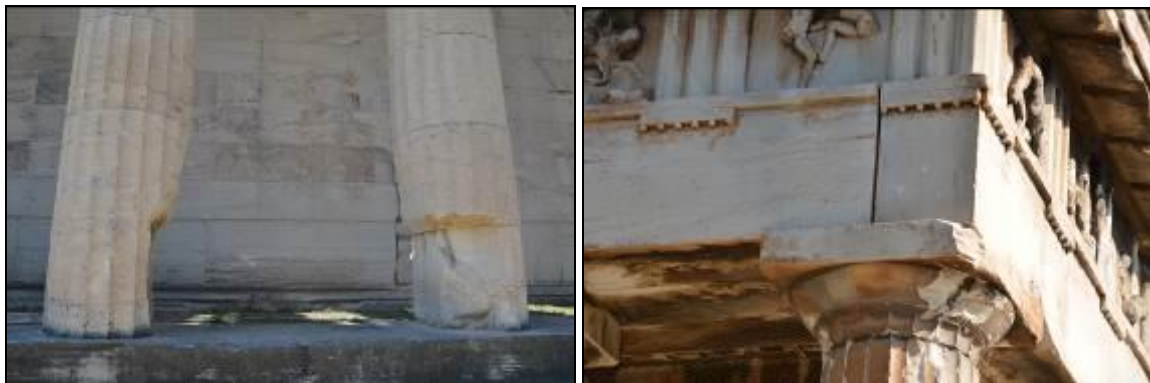
Figure 3. (a) Cutoffs of the lower drums of the columns at the north side of the temple; (b) opening of the joints of the architraves at the corners of the temple.
