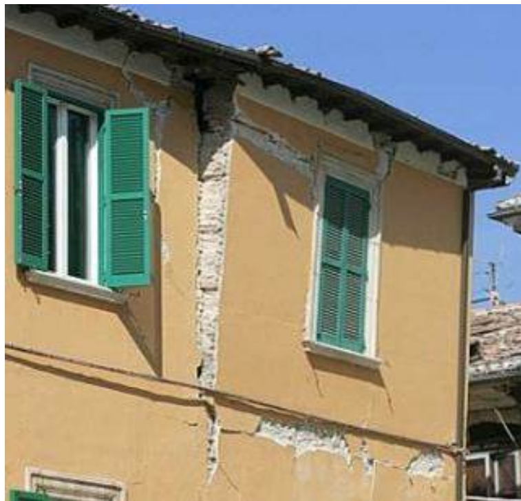
Figure 1: Out-of-plane damage of a facade segment, L'Aquila (central Italy) 2009.
