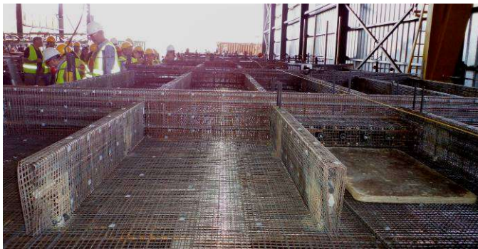
Figure 11a. Reinforcement of the pre-cast parts of the hollow roof
