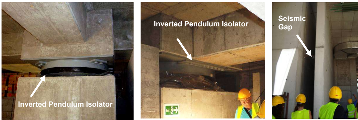
Figure 2. The base isolation system of the Stavros Niarchos Cultural Center main building formed by inverted pendulum bearings.
