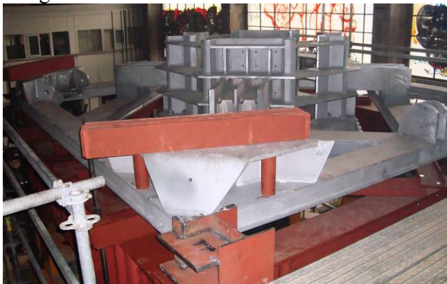
Figure 13. The 3-D polygonal steel rigid frame of a suspension unit. The 4 strong corners of this frame that represent the connection areas to the hollow suspended roof are also visible.
