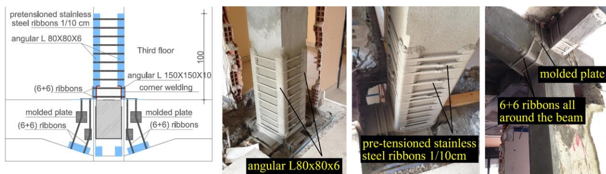
Figure 8 Strengthening of beam-column joints of the last elevation through pre-tensioned stainless steel ribbons
