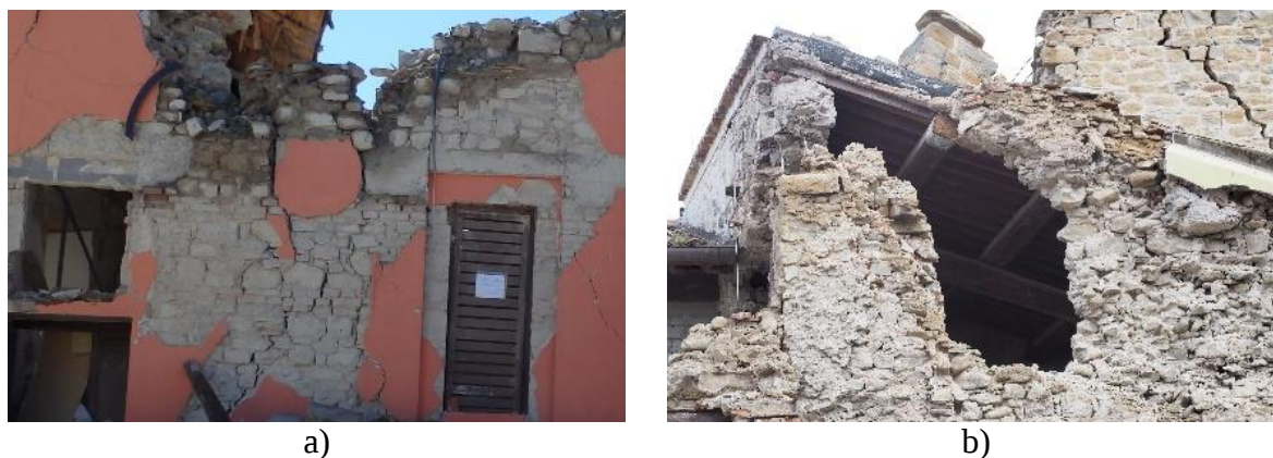
Figure 3: Details of the M2 and M3 masonry types in Amatrice
