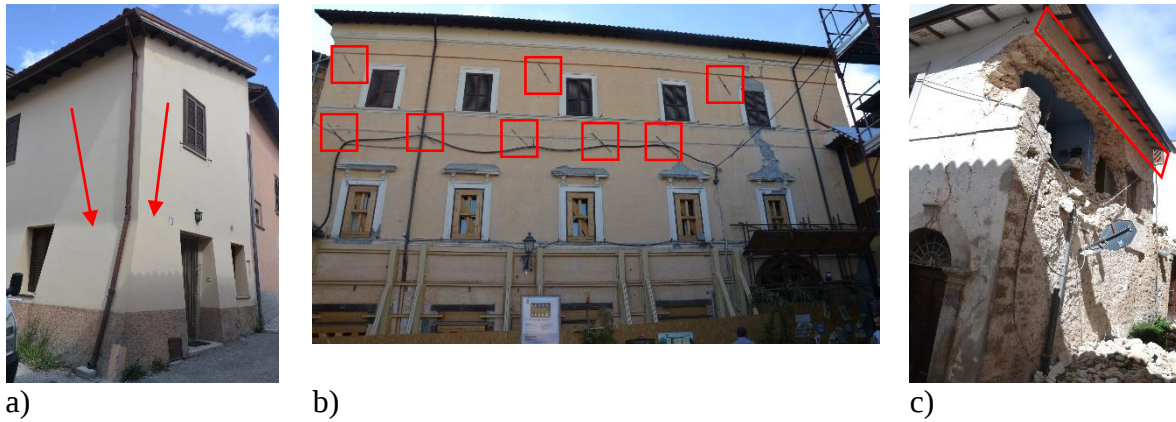
Figure 5: Restraining elements observed in Norcia: a) buttresses, b) ties o c) concrete ring beams
