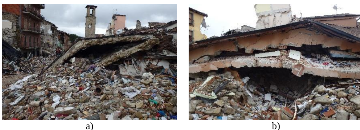
Figure 4: Details of the concrete slabs observed in Corso Umberto I – Amatrice
