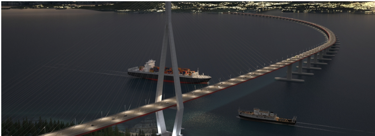
Figure 1: Floating bridge crossing the Bjørnafjord
