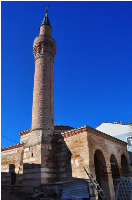
(a) North-East façade
