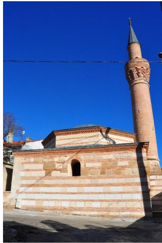
(b) South façade
