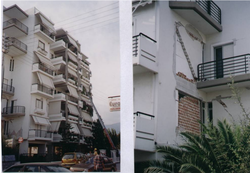
Figure 3. Relatively new unreinforced clay masonry infills at the façade of a multi-story reinforced concrete structure. These masonry infills became unstable and collapsed.
