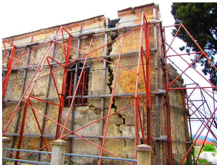
Figure 2. Old stone masonry church sustained heavy structural damage during the 2014 Kefalonia, Greece, earthquake sequence
