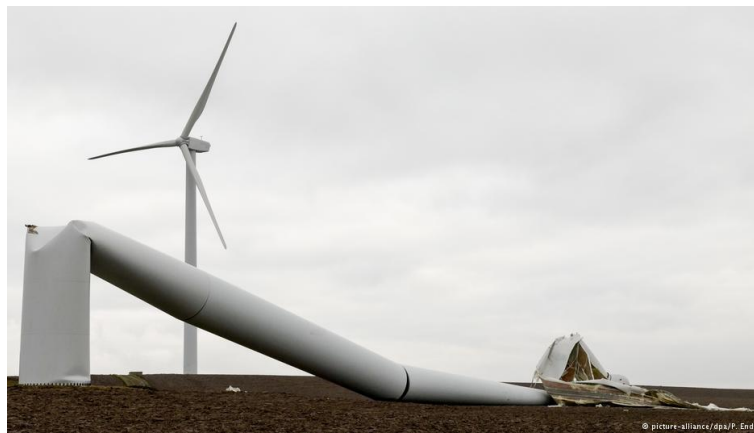
Figure 1: Collapsed wind tower [18]
