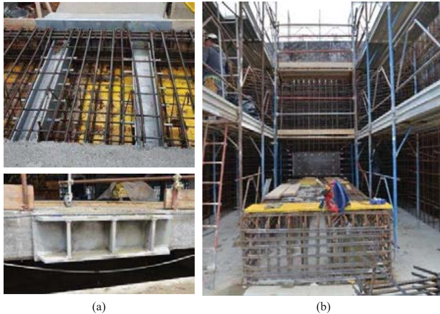
Figure 5: Reinforcement details of the building tall beam (a) and the reaction walls (b).
