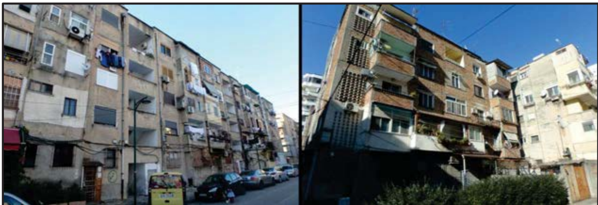
Figure 8: Undamaged multi-story masonry structures in Durrës.
