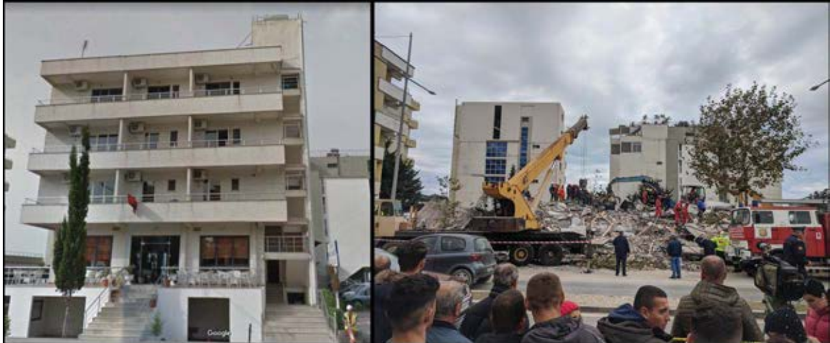
Figure 13: 4-story collapsed building in Durrës (Left photo: [27], Right photo: courtesy of C. McKenney [28]).
