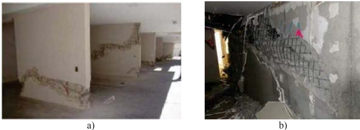
Figure 1: Observed damage to RC structural walls in a) the 2010 Chile earthquake [3] and b) the 2011 Lyttleton earthquake, New Zealand [2].
