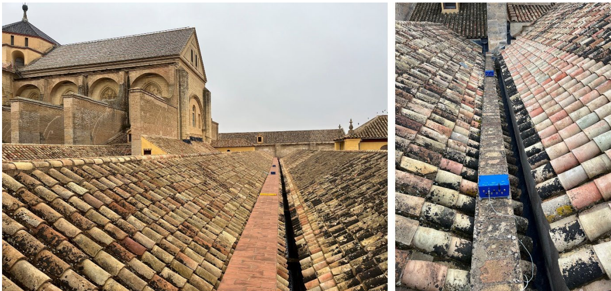
Figure 4: Location of the accelerometers in the arcades for the OMA.
