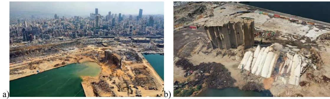
Figure 1: a) The damaged grained Beirut port silos, after August 4, 2020 blast [24] and b) The collapse of the North block silos [25].
