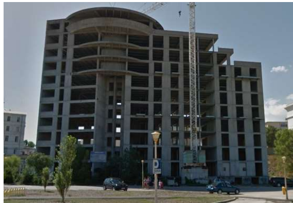
Figure 1: View of the existing building
