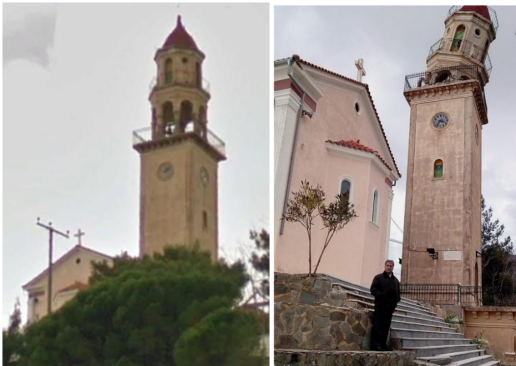
Figure 9. The bell tower at Kourouklata priot and after the earthquake sequence of 2014.
