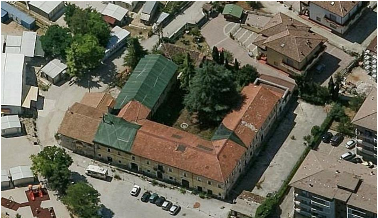
Figure 4 – S. Antonio church and masonry buildings aggregate
