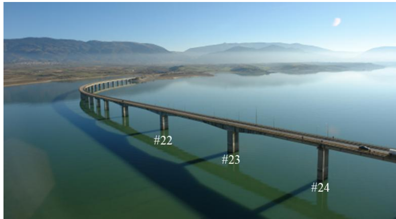
Figure 1: Polyfytos Viaduct, piers #22 and #24 (Gefyra Polyfytyou Servia, by Wikiphysicsgr, originally uploaded on 4 June 2011 to English Wikipedia. Transferred to Wikimedia Commons by Ronhjones. Available at: Wikimedia Commons. Licensed under CC BY-SA 3.0).
