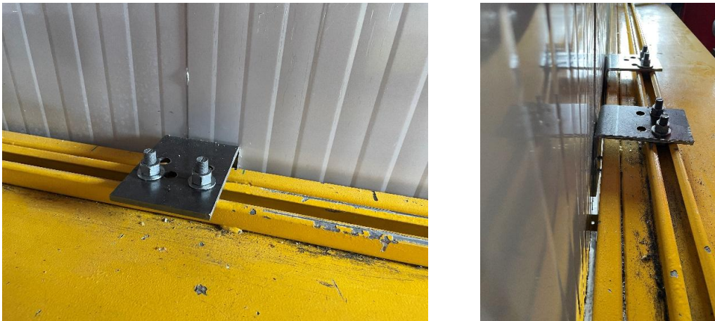
Figure 4: Panel connections (L-shaped steel bracket).
