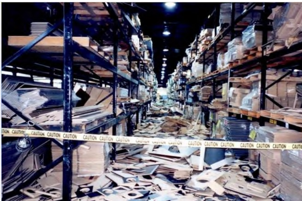
Figure 1 Damage to inventory on industrial storage racks in the 1994 Northridge Earthquake [2].
