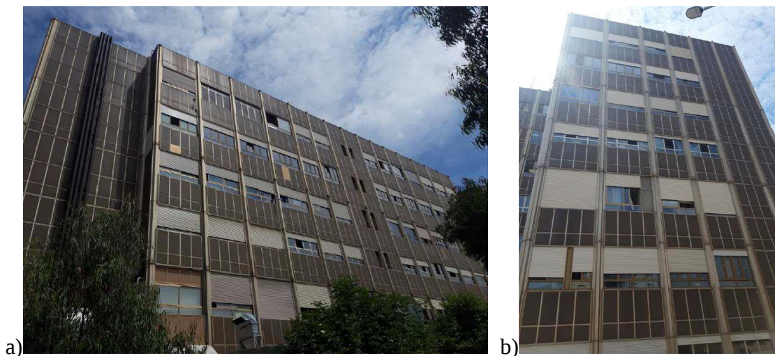
Figure 1: External views: a) South Side; b) North Side.
