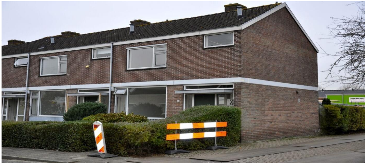
Figure 1: Typical modern masonry building with gable walls.
