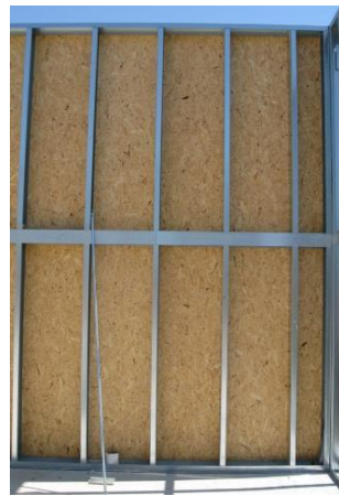
Figure 1: Typical shear wall with OSB panels.
