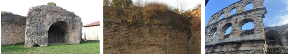
Fig. 2 Data acquisition in historical building wall
