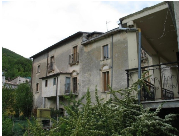
Fig. 2 South-east longitudinal façade of the masonry aggregate (Image courtesy of Prof. Luigi Sorrentino, DISG, Sapienza University of Rome)
