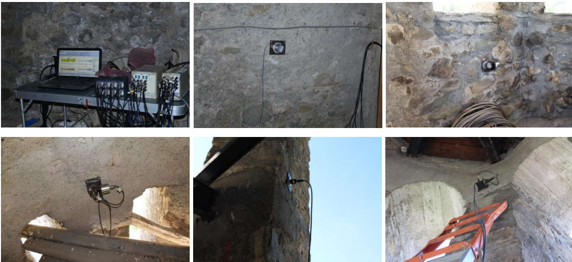
Figure 3: Measuring station and some positions of accelerometers.
