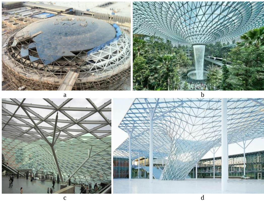
Figure 2: Gridshell examples: a) ‘The Orchard’ Doha Airport, b) Singapore Changi Airport, c) Złote Tarasy Warsaw, d) Fuksas Trade Fair
