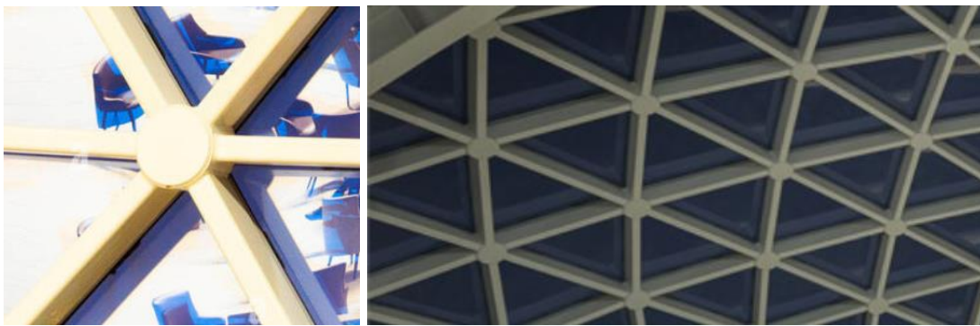
Figure 1: Fiumicino Terminal gridshell
