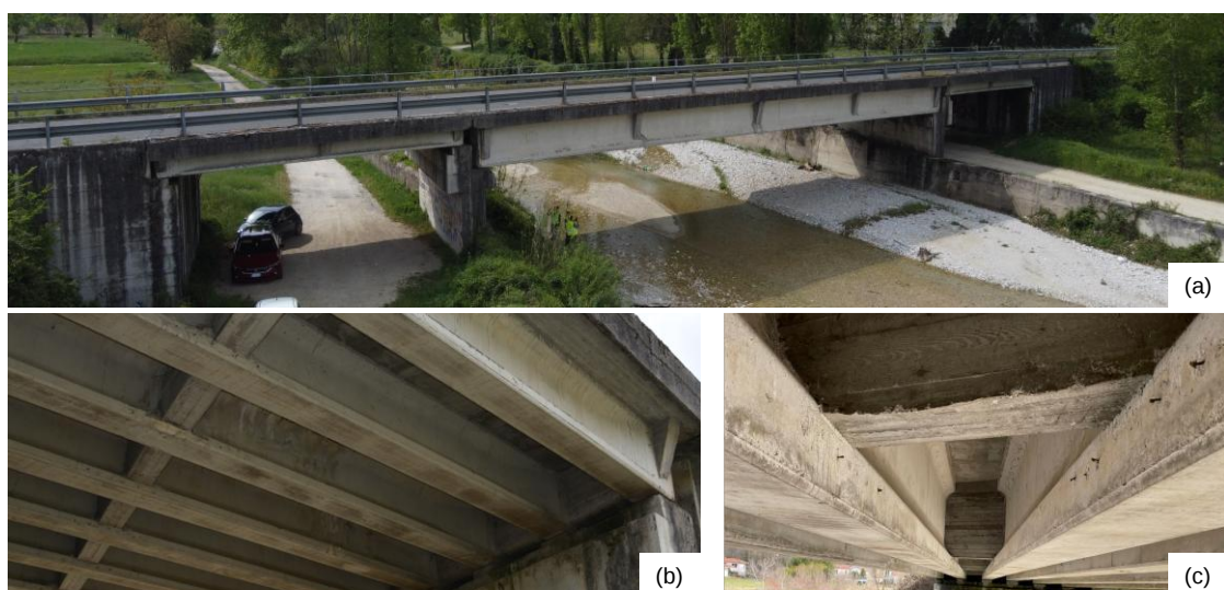
Figure 1: Bridge over the Mollarino torrent – Atina (Frosinone, Italy): overview (a), beams layout of lateral spans (b) and central span (c).
