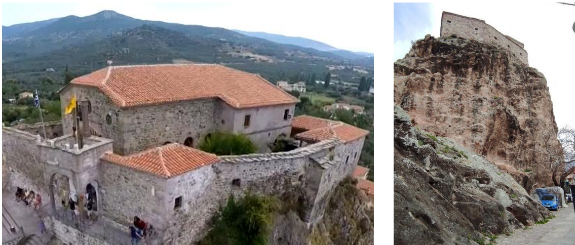
Figures 1 and 2: Temple of the Dormition of the Theotokos, perimetric fortification walls and rocky outcrop.
