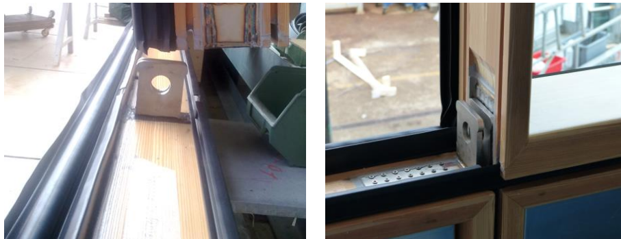
Figure 4: Bespoke spigots at the corner of the units.
