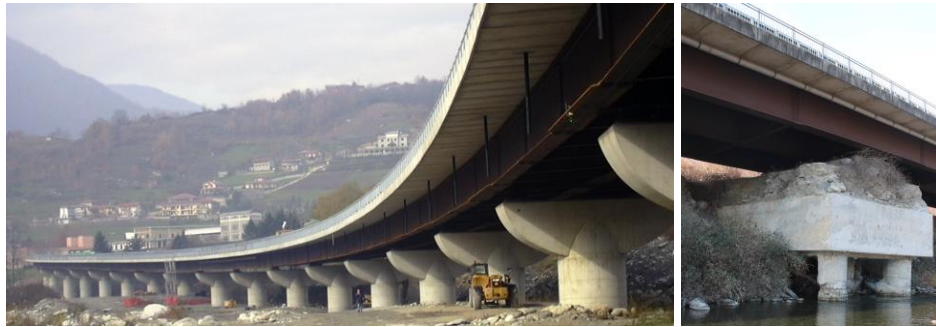
Figure 1: left, view of the Inverso Pinasca Bridge during construction (2004; Image courtesy of Seteco Ingegneria s.r.l.). Right view of current scouring conditions at pier P09 as of June 2023.
