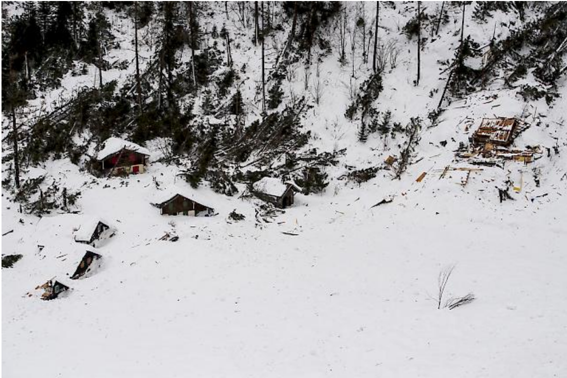
Figure 1: On March 8, 2017 a snow avalanche destroyed several chalets at the Swiss village of Salvan, Canton Wallis. Impact pressures were higher than 30 kPa. The air-blast from the avalanche blew down several trees behind the buildings. The building on the right was completely destroyed. The picture appeared in the Walliser Bote on March 8, 2017.
