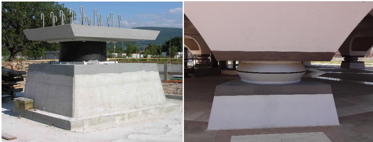
Figure 6 Support of an isolator during the construction and after its completion
