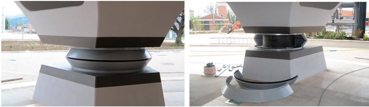
Figure 7 SI-S 1000/240 elastomeric isolator installed
