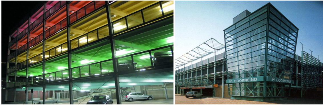
Figure 1: External views of typical steel framed open car park structures.
