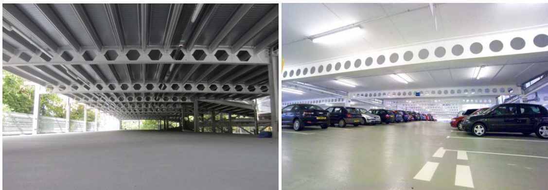
Figure 2: Internal views of typical steel framed open car park structures.
