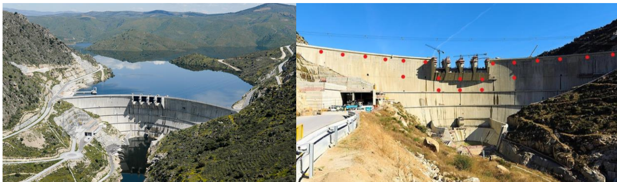
Figure 1 – Baixo Sabor arch dam: a) aerial view (on the left) [7]; b) position of accelerometers marked with red dots (on the right)
