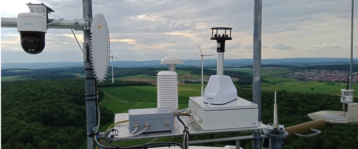
Figure 4: Overview of the roof installation - environmental measurement and antenna setup
